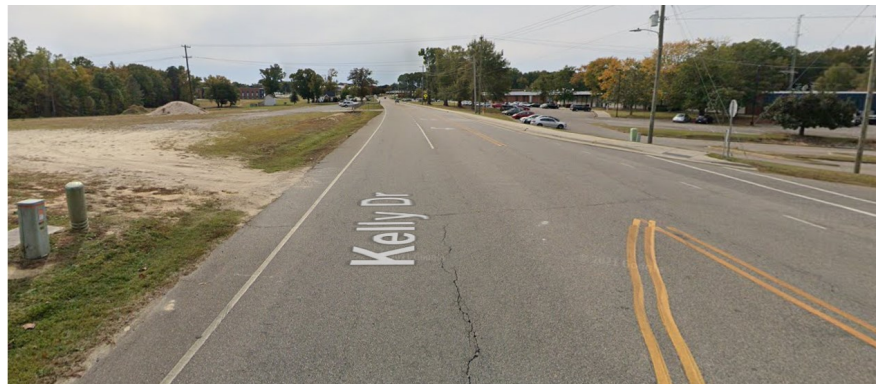
Current conditions on Kelly Drive In the vicinity of the proposed roundabout
