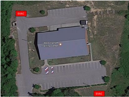
West Harnett Training Center (0060)
